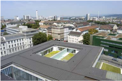
View from the roof of the Kantonsspital
